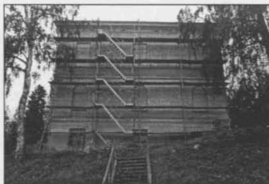
Fasaden under restaurering
